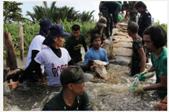
The Thai military and volunteers work to repair a leak in a dyke in Bangkok, 31 October 2011.
