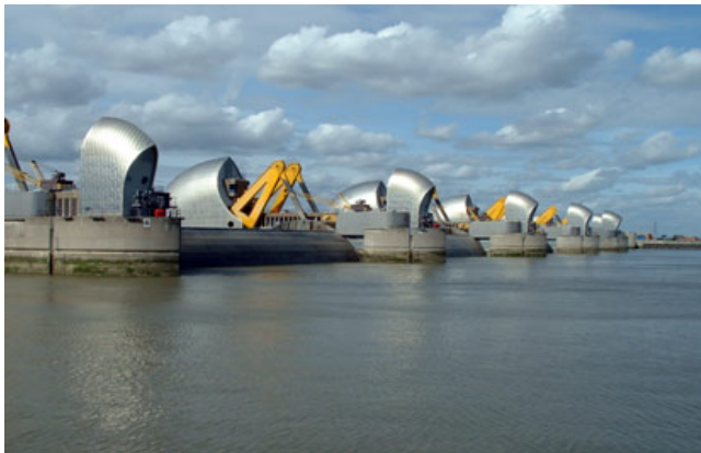
The Thames Barrier in London for flood/ surge protection
